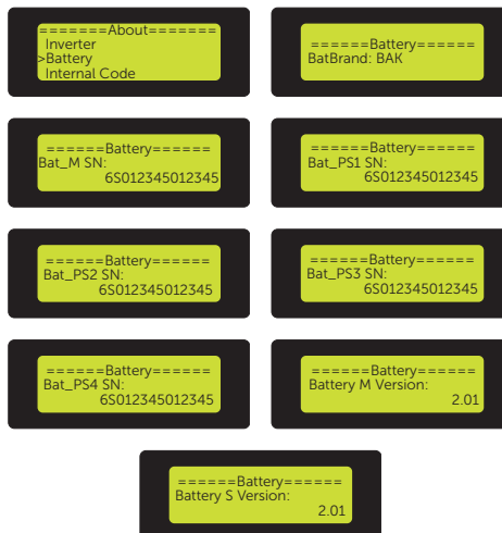
Figure 9-108 Displaying the battery information
